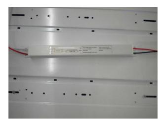
Step 3. According to the schematic wiring diagram, connect the wire of L(red wire), N(white wire) of the LED driver to the supply wire of the luminaire, connect the output wires of LED driver to the wire of the lampholder at both sides.
